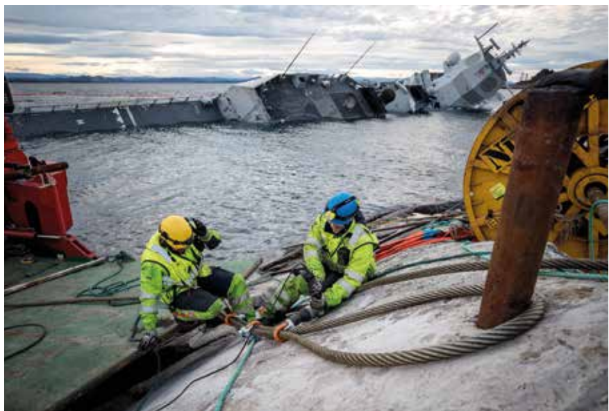
On 9 November, the frigate was secured with powerful steel wires and bolts to the rocks onshore.
